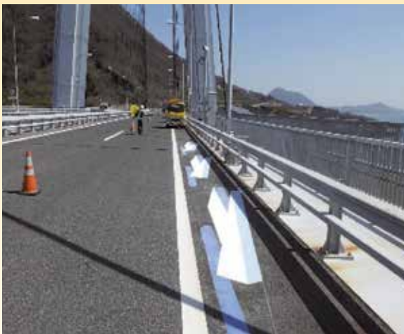
Three-dimensional arrow road surface signs using optical illusion
