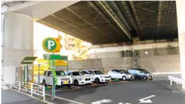
Parking lots (under elevated structures)
