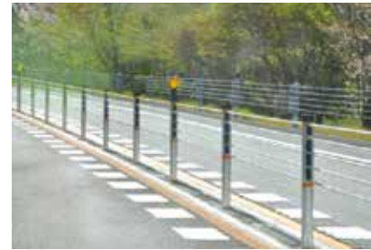
Installation of wire ropes
