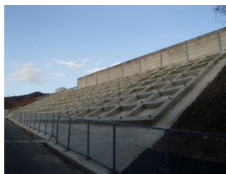
(盛土のり面補強の状況)
